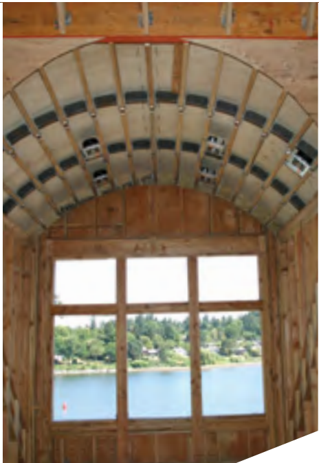
PN3MR 3-inch, NON-IC low-voltage housing platforms install easily into the tight framing that defines the barrel vault of this complex gable.
