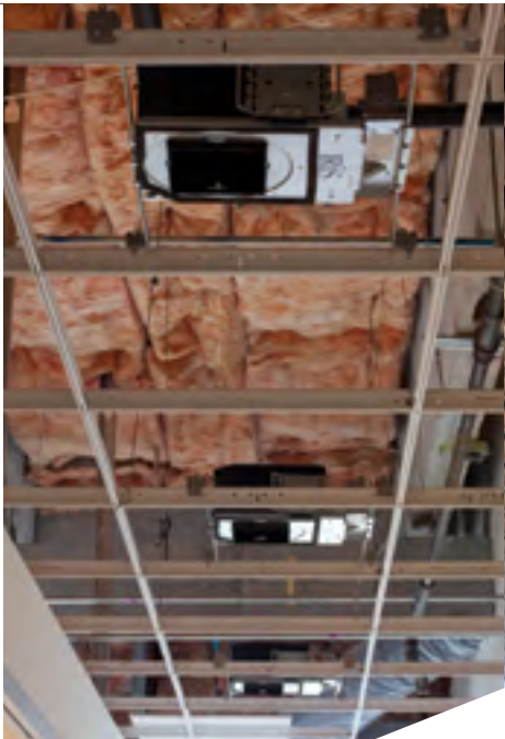
P406TAT 4-inch, square housing platforms adjust and lock into position on rigid bar hangers which clip directly to T-grid ceiling.
