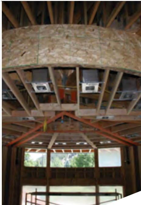
P3MR 3-inch, IC low-voltage housing platforms adjust and lock into position on rigid bar hangers, allowing accurate alignment in this bold residential space.
